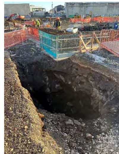
Figure 11: Unexpected voids in basalt
