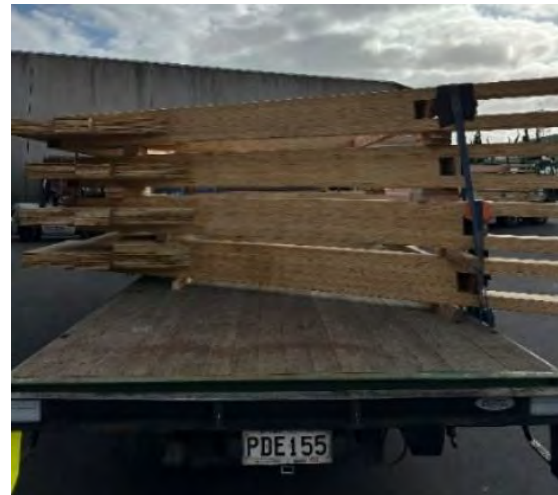
Figure 9: (Left) Diagrid prefabrication, (Right) Diagrid loaded for delivery
