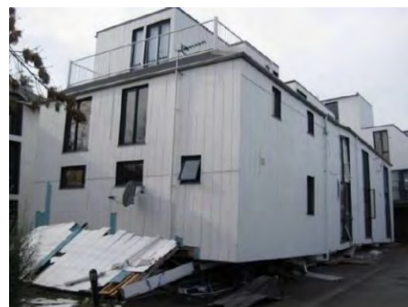
Figure 1: a) Case study 1 before and b) after 22 nd of February 2011, c) Case study 2 immediately after the earthquake and d) soft storey collapse due to wind several days later. (Buchanan et al. 2011).
