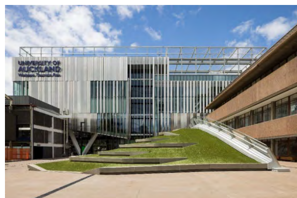
Figure 3 - Plaza mound directly above the pool hall, formed by cranking of the box girders.
