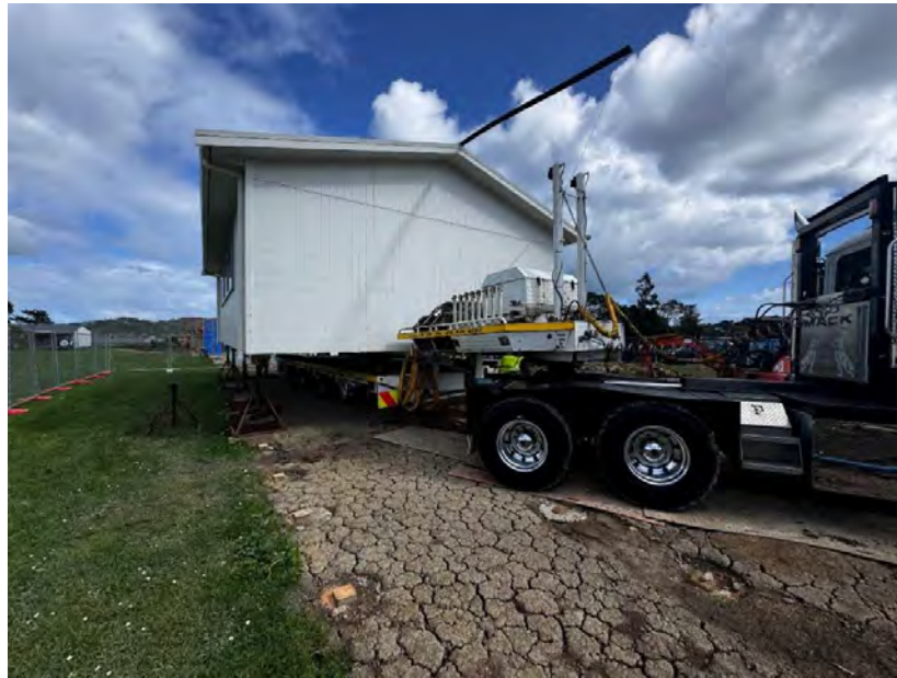
Figure 4 - Existing A-line classroom at Waiheke High School being prepared for relocation to Massey High School
