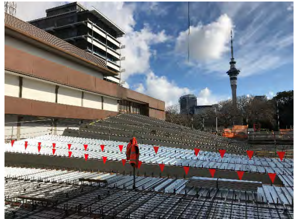
Figure 13 - Metal-deck placed for 180mm slab.
