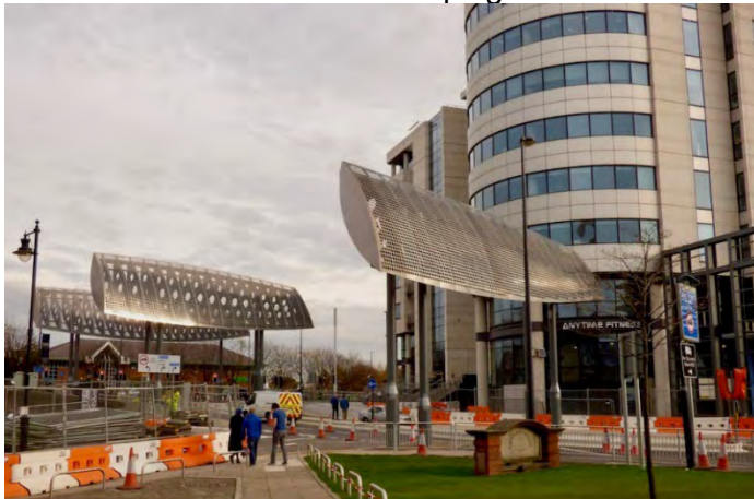
Figure 1: Bridgewater, Leeds, mitigations required to decrease wind related hazard around development.
