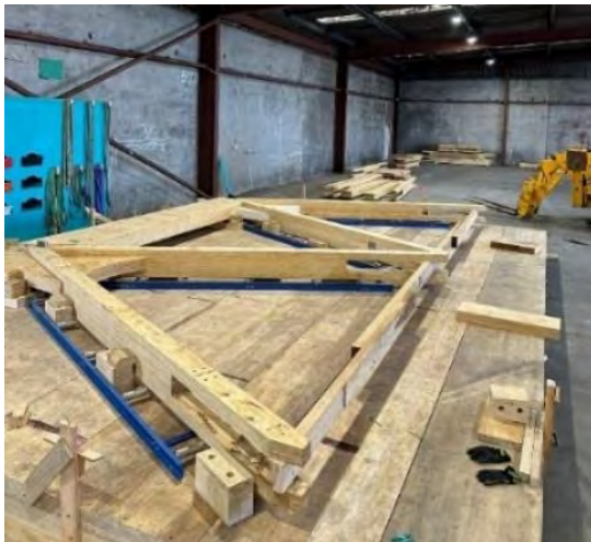
Figure 9: (Left) Diagrid prefabrication, (Right) Diagrid loaded for delivery
