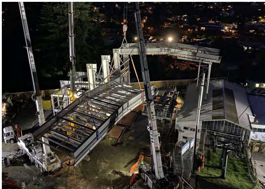
Figure 8: Construction of the new Bottom Terminal Building over the existing Bottom Terminal.
