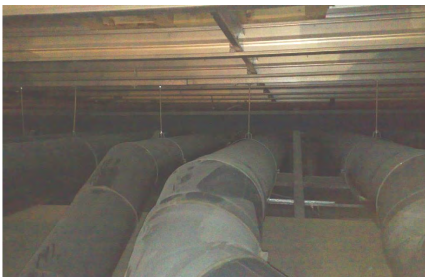
Figure 7: Fume extracts in Alan MacDiarmid running over the "Ghost Floor" (bottom of image) below lightweight roof
