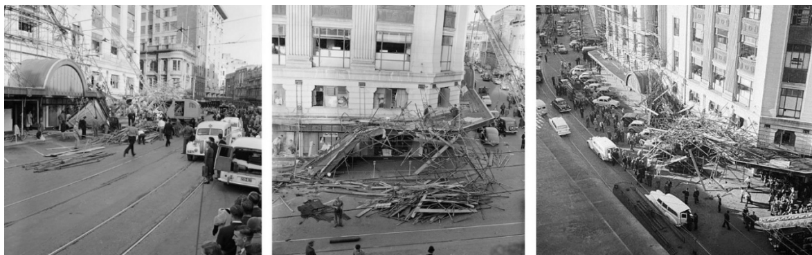
Figure 2: Collapse of the scaffold – DIC Building, Wellington. (source: Alexander Turnbull Library)
