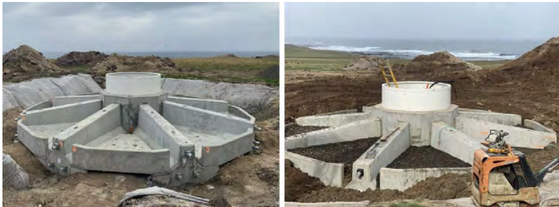
Figure 4: On-site assembly photos of the foundation structure.
