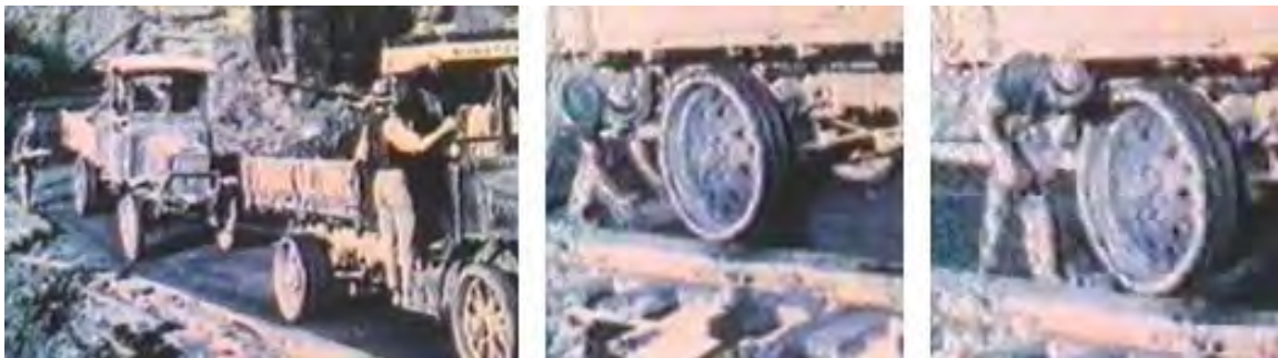
Figure 1: A worker dangerously chocks the wheel of a brake-less truck as it is towed up a slope during the excavations for the construction of the Civic Theatre. (source: TVNZ)
