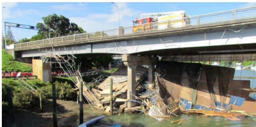
Figure 4: Scaffold collapse – Panmure Bridge – Auckland. (source: RNZ News)
