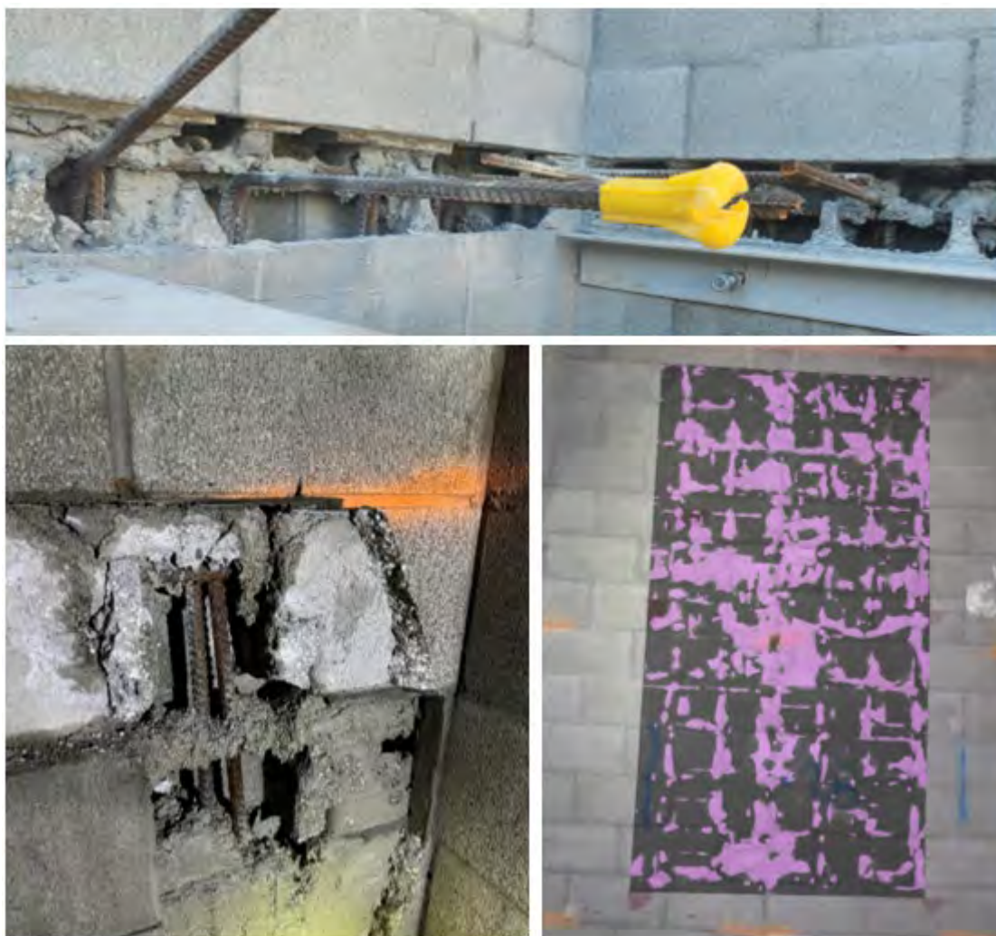
Figure 2: Voids found via intrusive inspection in RCM wall. This wall was constructed in 2024 with construction monitoring undertaken by structural engineers. Note the right image shows Ground Penetrating Radar scans of areas of 'low density'. A skilled scanner is needed to interpret these results as not all highlighted areas are voids. Photo credit: Beca Ltd.
