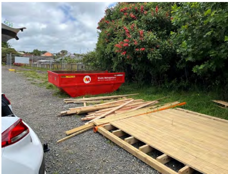
Figure 3 - Deck Module constructed off site prior to installation
