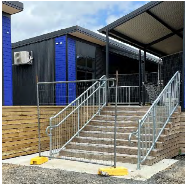
Figure 2 - Proprietary Moddex barrier and handrails installed on stair
