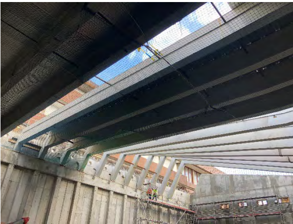
Figure 12 - Box girders installed.
