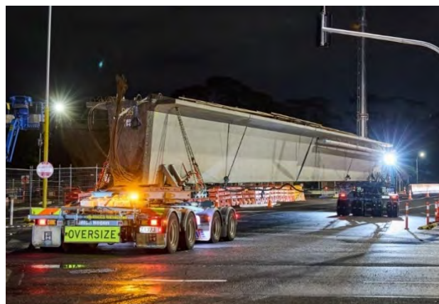
Figure 6: Super T beam delivered to site with handrails, edge forms and drainage installed
