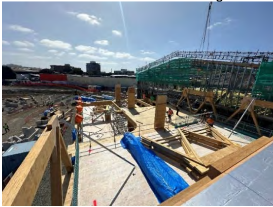
Figure 10: (Left) Lineal building construction and installed membranes, (Right) Façade following behind structural erection
