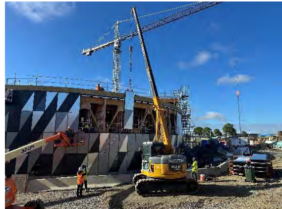
Figure 10: (Left) Lineal building construction and installed membranes, (Right) Façade following behind structural erection
