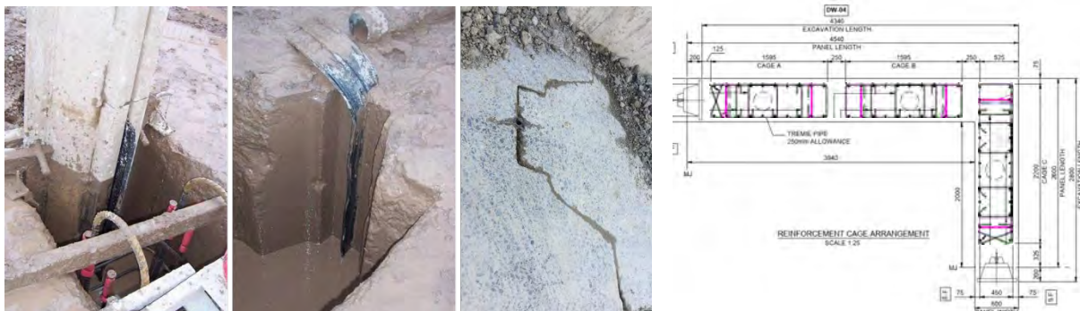
Figure 7: Diaphragm wall inter-panel joint & cage layout
