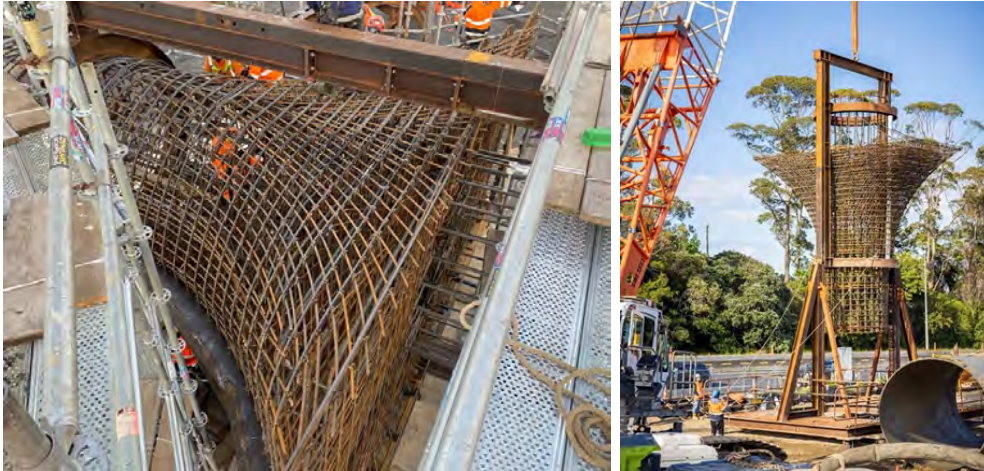
Figure 4: Off-site fabrication of pier flare and plunging operation
