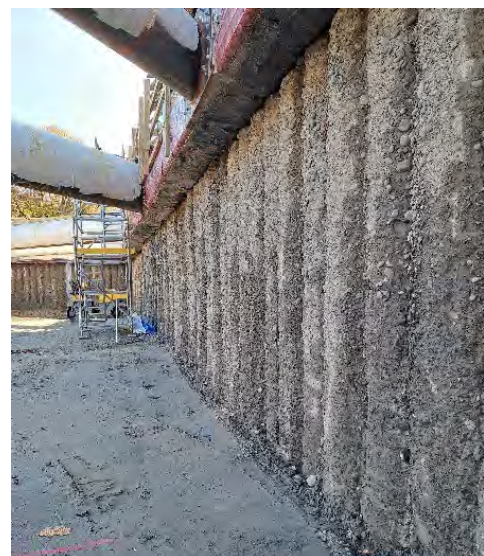
Figure 5 Secant pile wall
