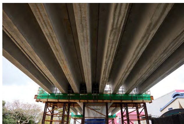
Figure 7: Superstructure falsework and steel diaphragm formwork between Super T beams
