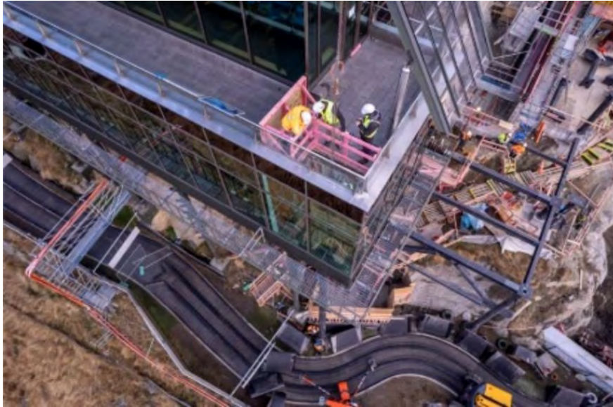
Figure 6: New Column being installed through existing live restaurant for the Extension structure
