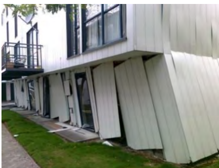
Figure 1: a) Case study 1 before and b) after 22 nd of February 2011, c) Case study 2 immediately after the earthquake and d) soft storey collapse due to wind several days later. (Buchanan et al. 2011).
