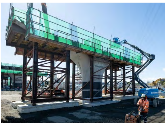
Figure 7: Superstructure falsework and steel diaphragm formwork between Super T beams
