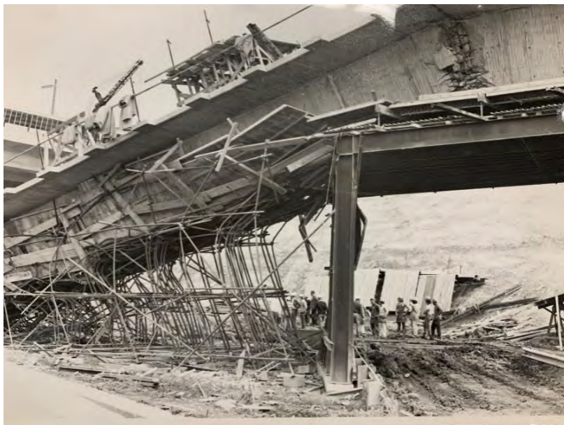
Figure 3: Collapse of Ramp A – Auckland. (source: WSP)
